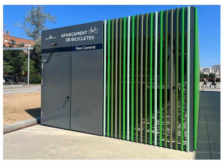
In Girona's Parc Central, next to the high-speed train station, the bus station and close to the Renfe train station, a parking area with a capacity for 70 bicycles has been installed. It is made of a metal structure based on coloured laminated profiles and is designed to be flexible so that it can be expanded or reduced, or moved to another location if required in the future..
