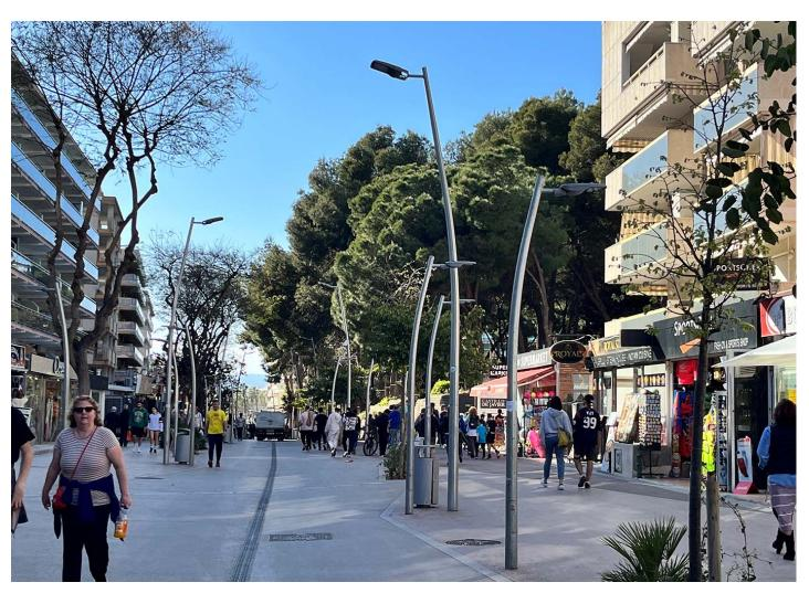
The coastal town of Salou has dozens of Ter lighting points installed on Carles Buïgas Avenue, with 7-meter Milan XXL RGBW floodlights and 4-meter Milan S40 luminaires. They are complemented by cylindrical poles. All the light points include LED technology and are controlled with the DMX remote management system through a touch screen to generate waves of colour on one of the main commercial arteries of the town.
